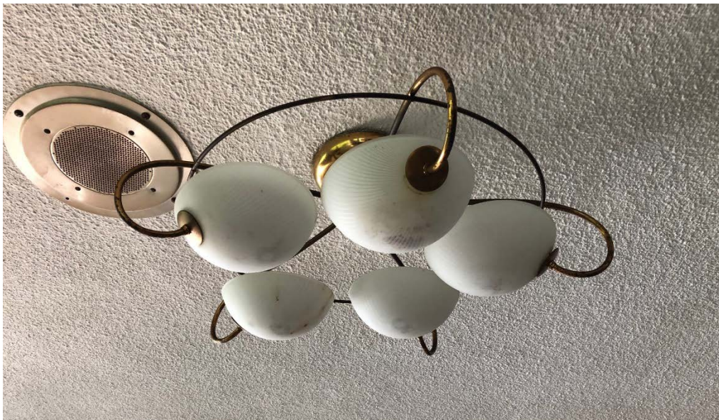
Lobby light fixture
