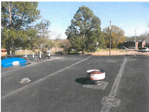
Flashing/Perimeter of the Roof (AS-03)
