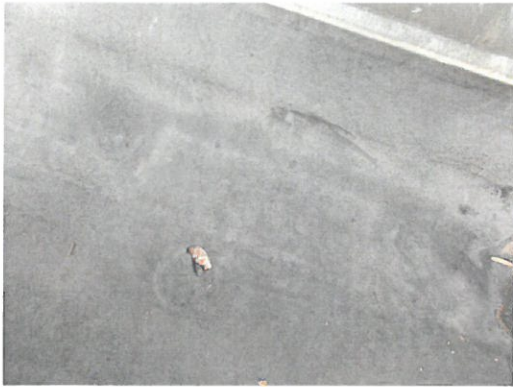
Roofing Material (AS-07)
