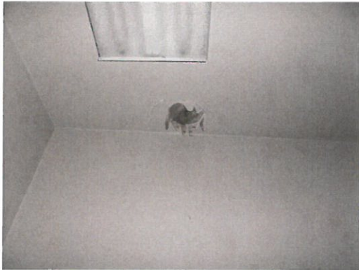
Sheetrock Ceiling/Kitchen (AS-01)
