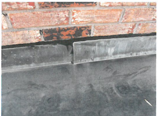
Mastic/Perimeter of the Roof (AS-06)
