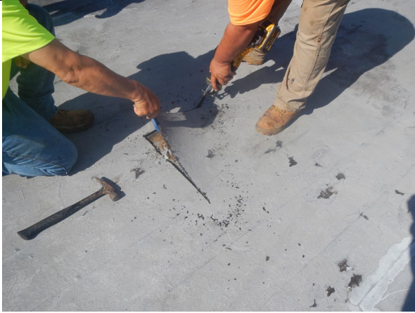
Removal of roof membrane (Roof A, LWIC)
