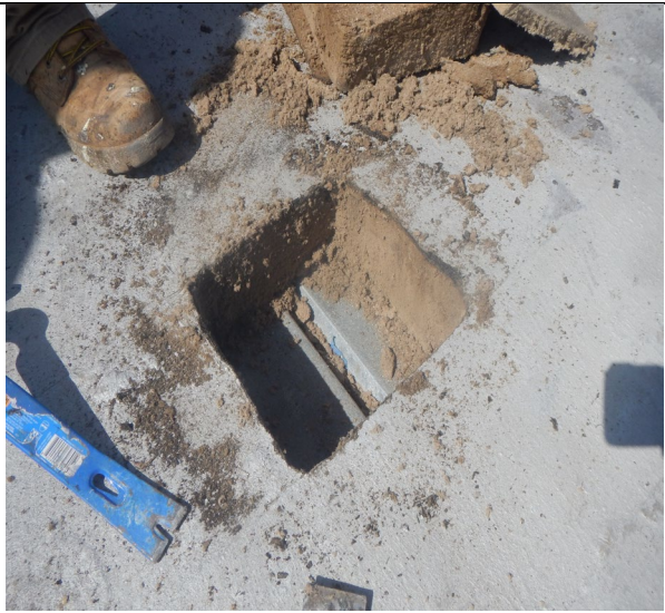
Metal deck at Roof B
