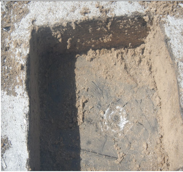
Core at Roof B
