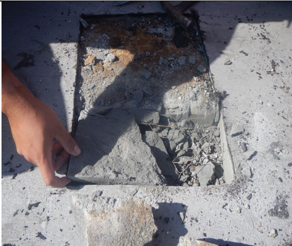
LWIC being removed
