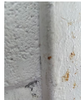
AS-09 Men's Visitor's Restroom Block wall
