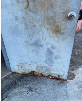
AS-01 Men's Bathroom Door
