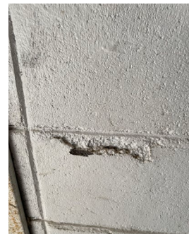
AS-06 Visitor's Concession Stand Block wall
